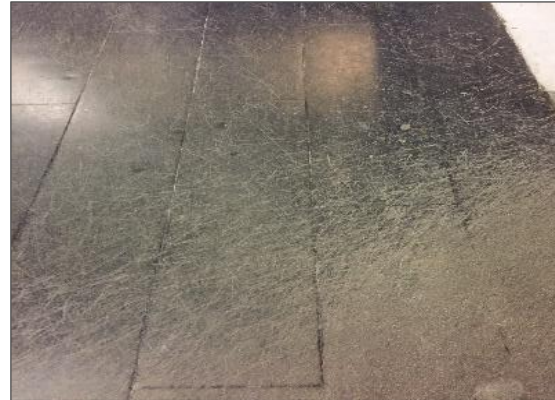
Photograph No. 5: Non-asbestos skate matting within the rink Loc.15 (Samples 0019A-C).
