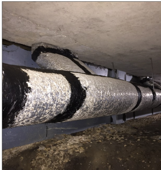
Photograph No. 25: Asbestos-containing black tar mastic on ducting within the south crawlspace (Samples 0009A-C).
