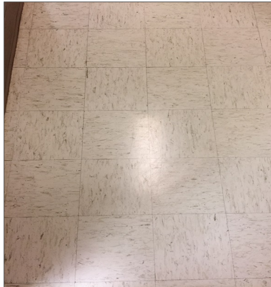
Photograph No. 16: Asbestos-containing vinyl floor tiles within the auditorium and adjacent rooms Loc.48 (Samples 0039A-C).
