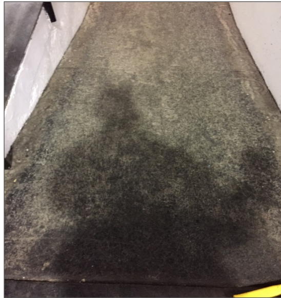
Photograph No. 6: Non-asbestos skate matting within the rink Loc.15 (Samples 0020A-C).
