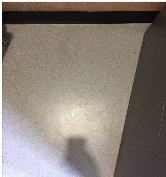
Photograph No. 9: Non-asbestos vinyl sheet flooring within the utility room Loc.53 (Rubber).
