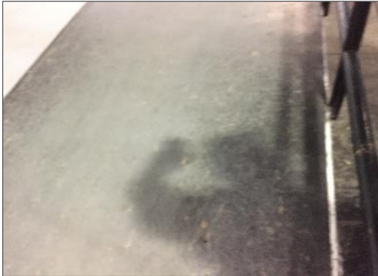
Photograph No. 4: Non-asbestos skate matting within the rink Loc.15 (Samples 0018A-C).
